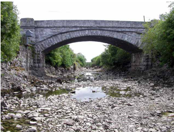
Carrownagower Bridge, Cong Canal
