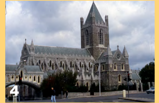
4 Christ Church Cathedral, Dublin: Limestone from Dublin & Meath with pale limestone and green slate from England
