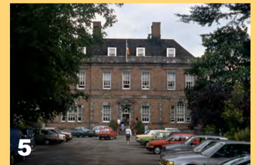
5 Cashel Palace, Co. Tipperary: Red brick
