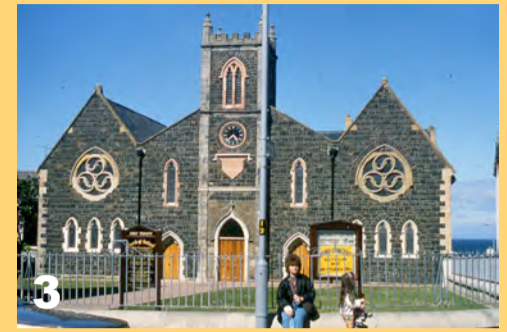
3 Holy Trinity Church, Portrush, Co. Antrim: Basalt walls and limestone around windows
